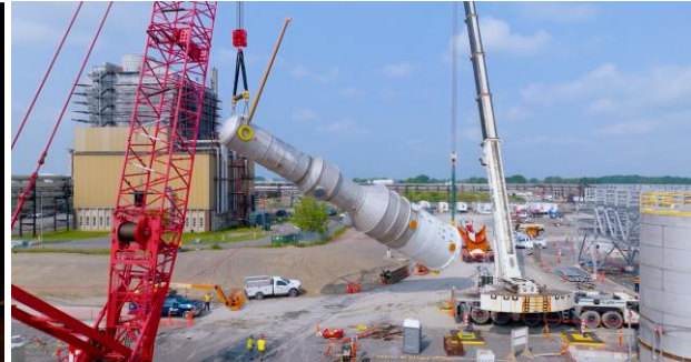
Aerial shot showing the safe delivery and installation of the largest piece of equipment at the Rochester Hub.
