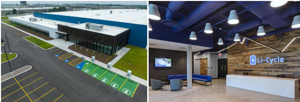
Completed Rochester Hub Warehouse and Offices.
