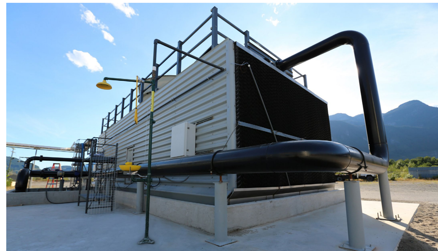
Carbon Engineering's pilot air contactor
